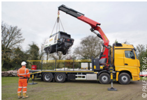
The mobile lift shows the main boom (red) and additional booms (black) which increase the reach of the crane.
